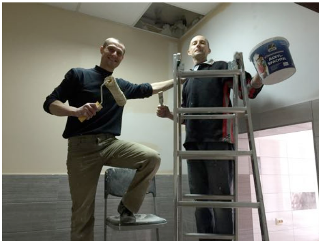
Reconstruction work in our new church building
